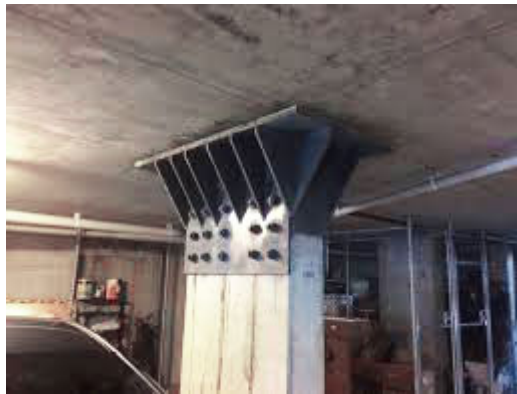
Figure: Additional shear reinforcement using steel bracket.
