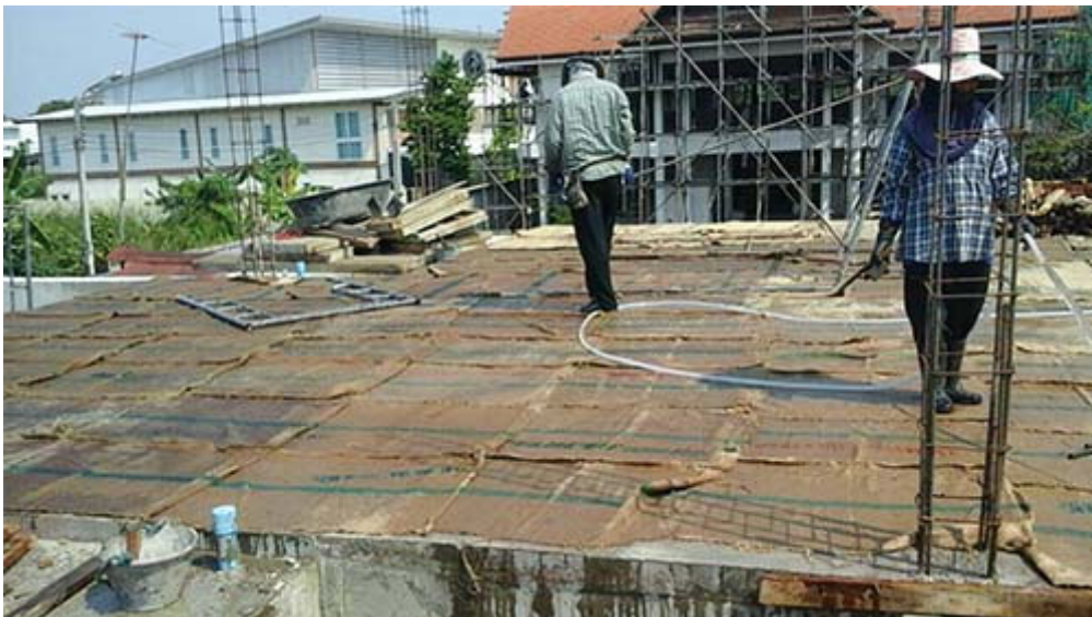
Figure exhibits curing through temporary bordering to retain water.
