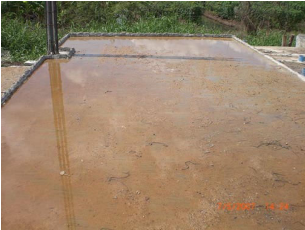
Figure exhibits curing through temporary bordering to retain water.
